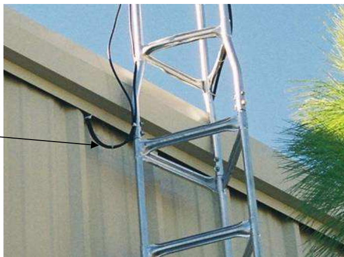
Figure 26. Creating a drip loop before entering the building
